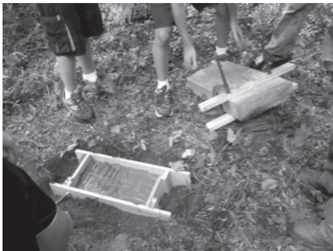
This photo shows a newly created rectangular wooden base filled with cement, and the stone which will be placed in it. To the right, bottom, the re-erected tombstone.
