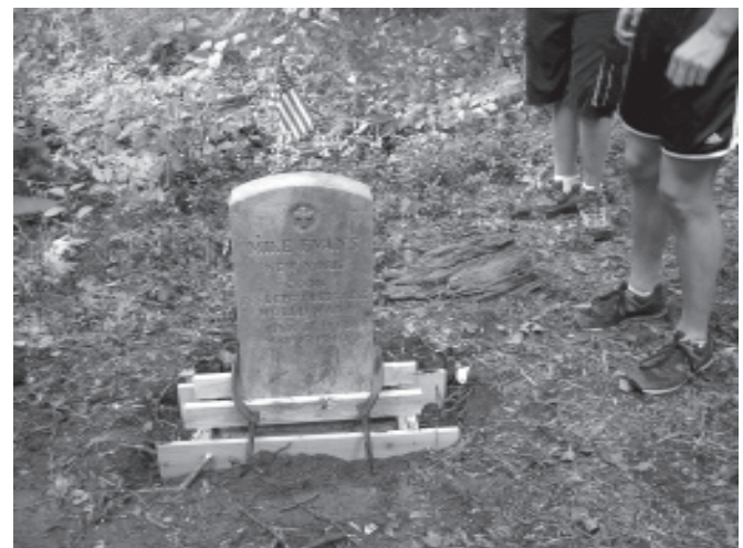
This photo shows a newly created rectangular wooden base filled with cement, and the stone which will be placed in it. To the right, bottom, the re-erected tombstone.
